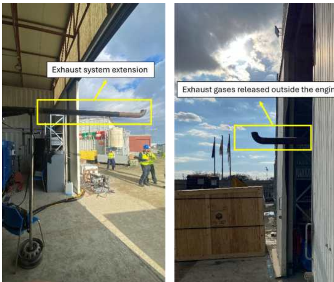
Figure 7: Extension of bypass pipeline outside the hangar.
