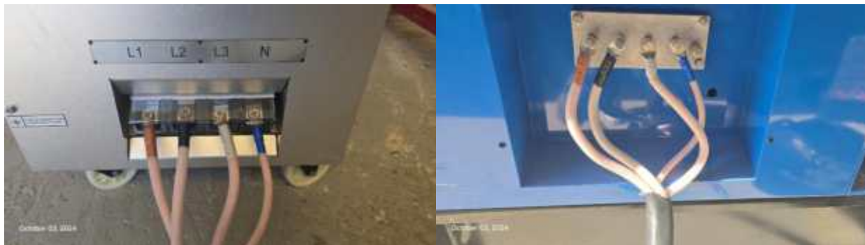
Figure 6: Left: Installation of wires with clamps the load bank. Right: Installation of wires with clamps the genset side. Note: Additional clamps were used for smooth integration.
