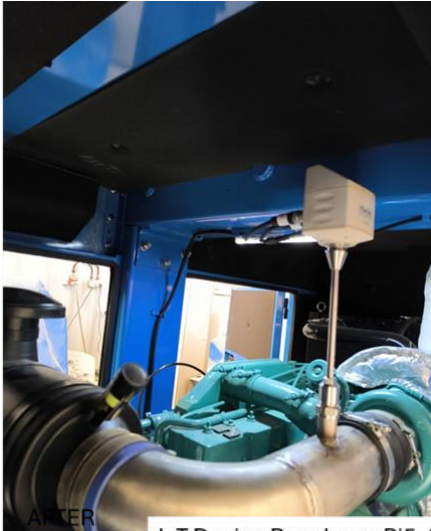
IoT Device Raspberry Pi5. Sensors with CanBus connectivity to IoT Network
